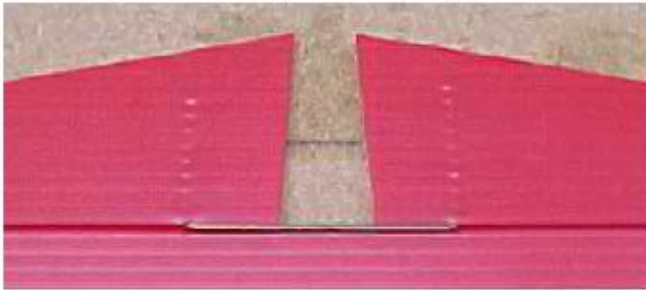
Elevator joiner close-up
